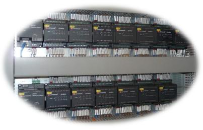
• PLCs have a large point capacity, allowing one controller to monitor and control large or multiple systems.
